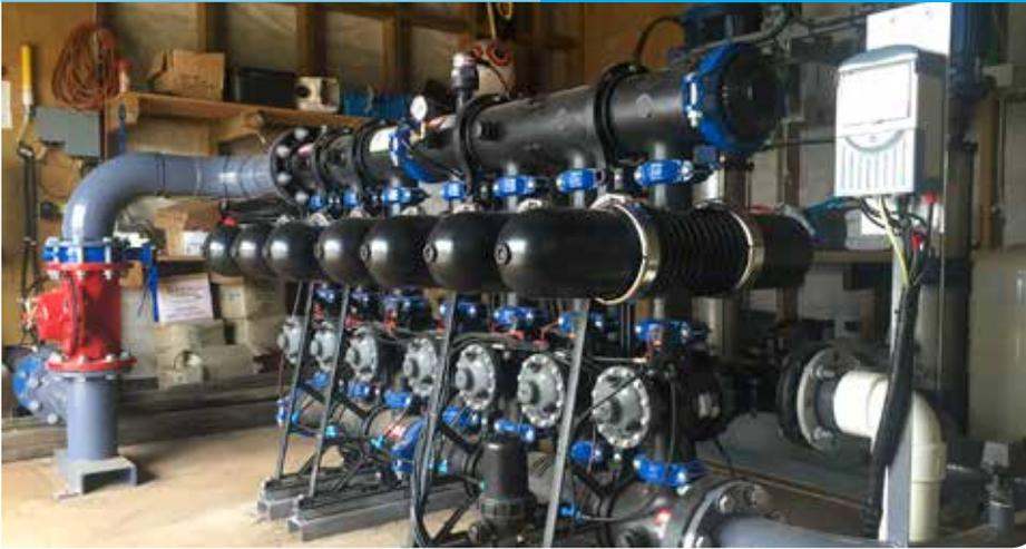
Liquid Action Ltd was asked to offer a filtration solution for a prominent vineyard in Marlborough's Awatere Valley. They in turn, asked our technical representative, Iain Holdaway, to design a new filtration system for the vineyard's man-made dam. The dam is filled by run-off, so water quality can be poor with lots of suspended solids, organic matter and debris.
